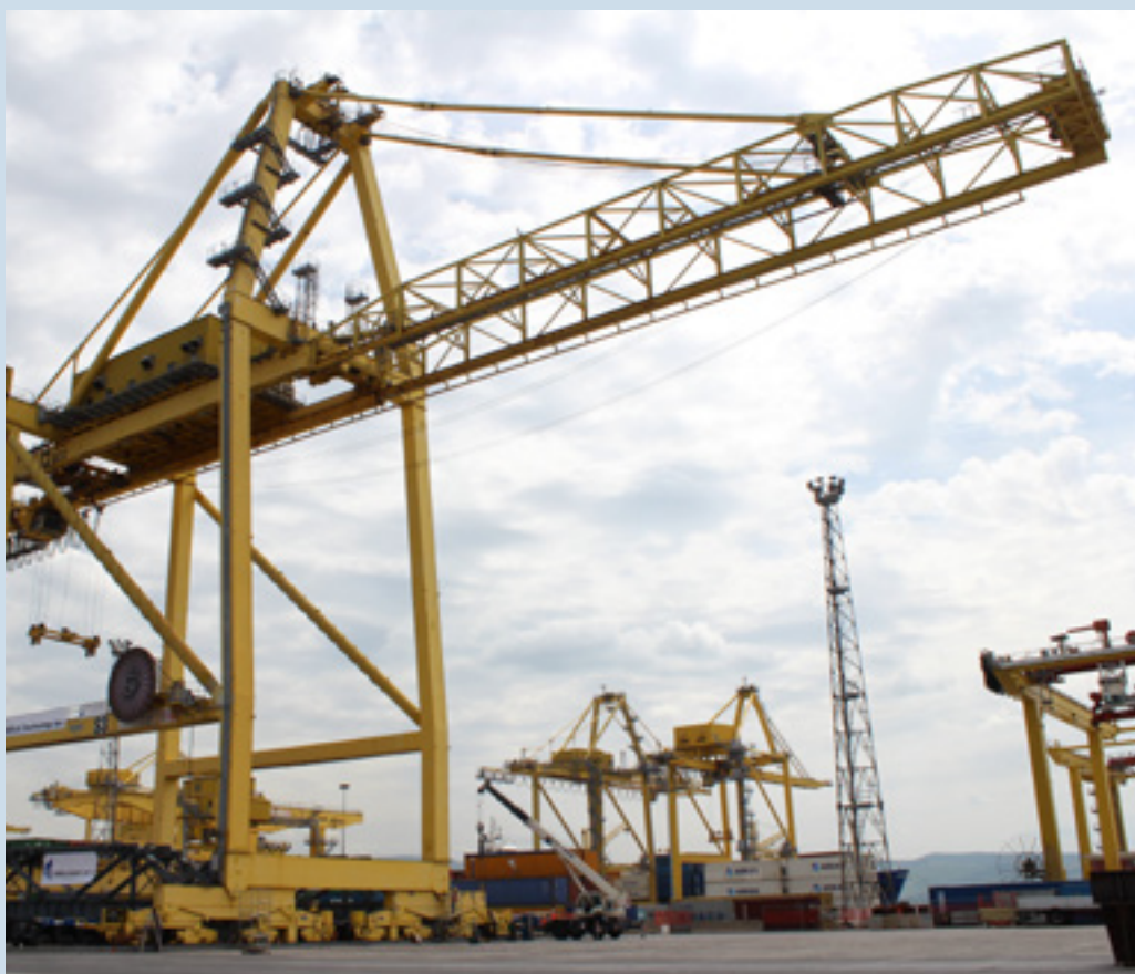
Molo VII, one of the cranes in operation
